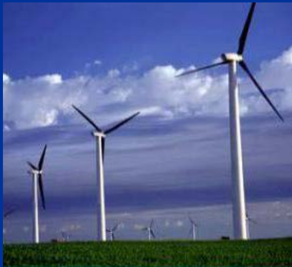
210 MW Lake Benton Wind Farm 4 cents/kWh
