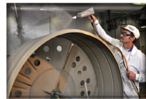
Restoration and Repair
